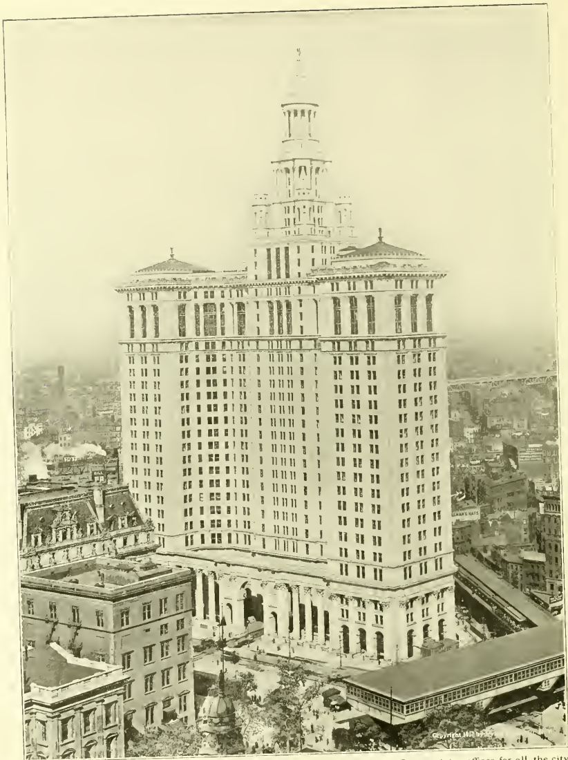
MUNICIPAL BUILDING—Facing City Hall Park at Park Row and Center Sts., contains offices for all the city departments and is the largest structure of its kind in the world. It is 34 stories, 580 feet high, including a 30 foot statue of Miss Civic Pride on tower. Foundation consists of 116 pneumatic caissons sunk 260 feet below water level. Total cost $13,000,000.
